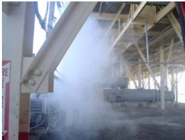
Nevada Geo Thermal Plant
